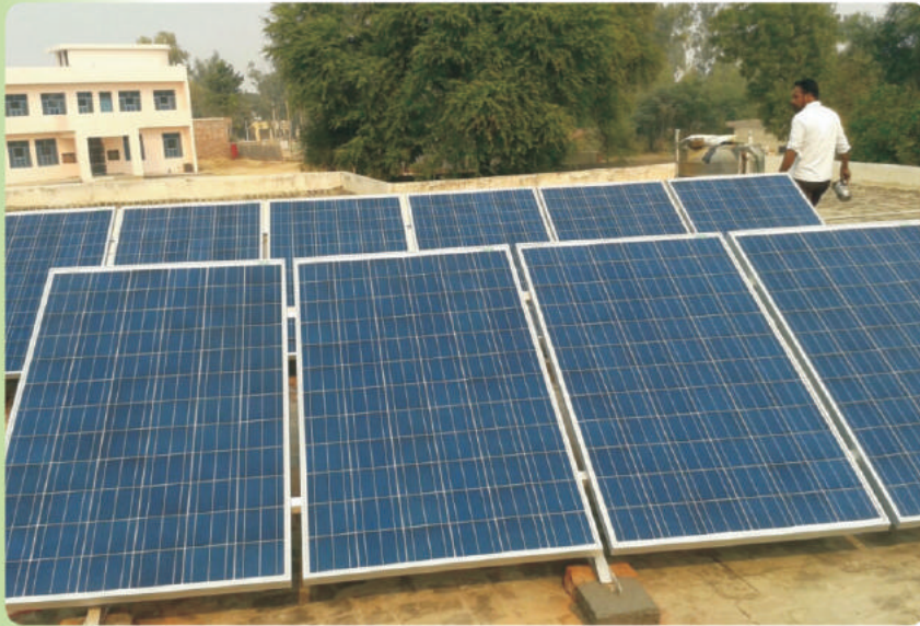
Grid Interactive Solar Power Plant installed at Punjab Police Station site inset view of Control Room
